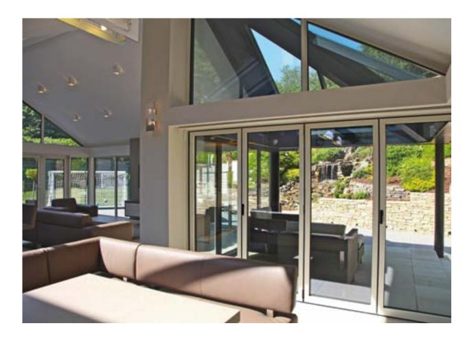
The Bi-fold doors incorporate multi-point security locking with bespoke hinges and full or half rollers. Shoot bolts, flush operating handles and euro cylinder options are also available for intermediate sashes. In addition, the door offers low U-values which can be further enhanced with a high insulation (Hi+) option of uniquely designed cellular foams which enclose internal cavities within the profile further reducing heat loss.
